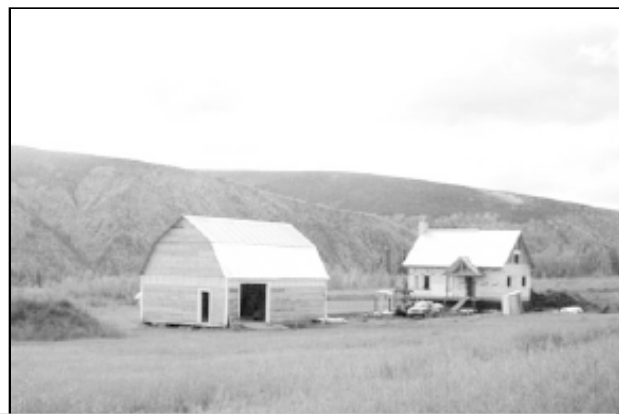
The Wilsons house and barn, showing the barn as it was before the twister demolished it.
