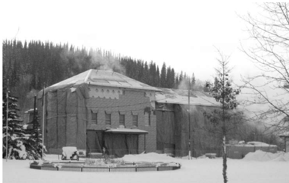
The new Dawson Hospital puffs out like a balloon as the contractor heats the interior shell for the workers.
