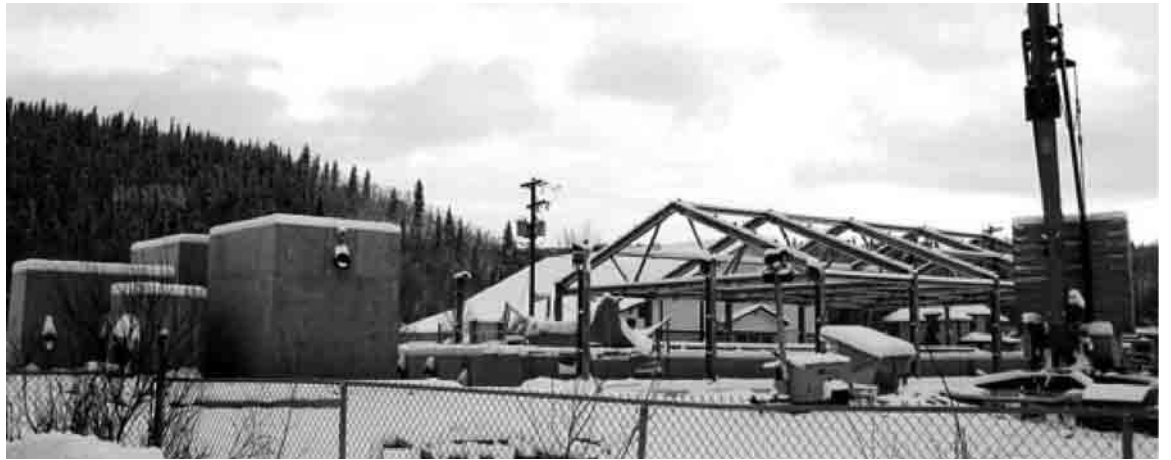
The Dawson City Wastewater Treatment Plant is under construction. The two concrete pillars at the left are the housings which contain the main and back-up vertical sewage treatment shafts at the heart of the Vertreat process.
