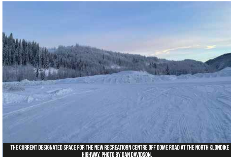
THIS IS THE OPEN SPACE BEHIND THE FAILED WASTEWATER TREATMENT PLANT, WITH THE BIOMASS FACILITY OFF TO THE LEFT IN THE PICTURE. PHOTO BY DAN DAVIDSON.
